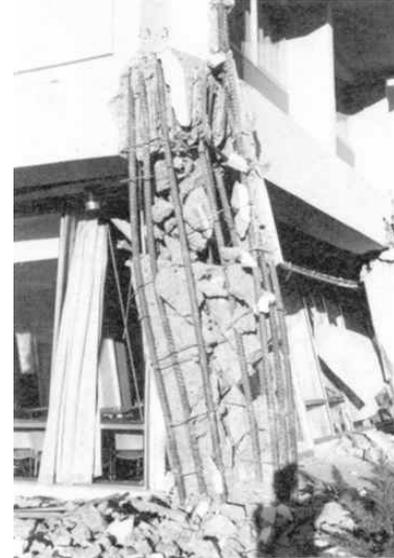
**(b) Brittle failure of a reinforced concrete column**
